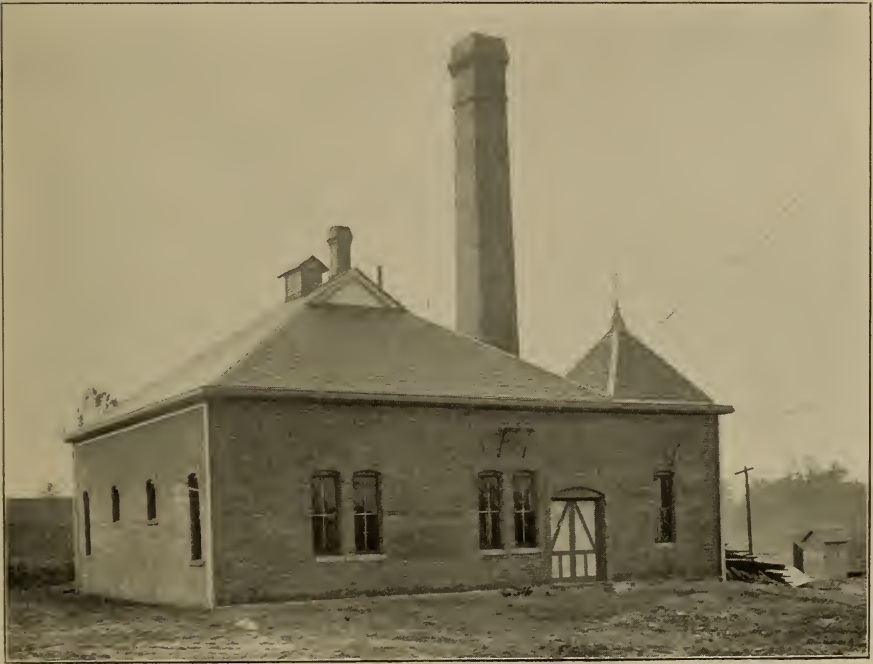
POWER HOUSE—LAWRENCEVILLE LIGHT AND WATER CO.
